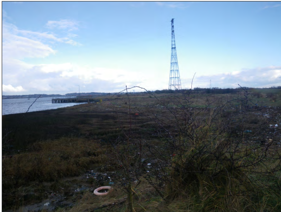
Plate 3: The Swanscombe Peninsula showing the super-pylon (WA754) and jetty (WA640)
