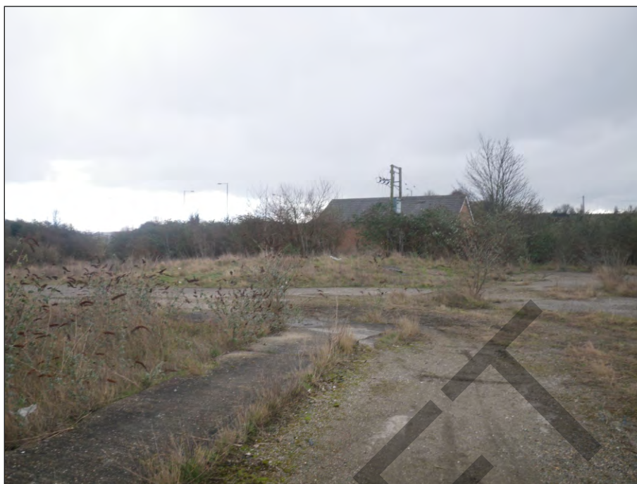
Plate 1: The concrete remains of the former Portland Cement Works within the Site, looking south
