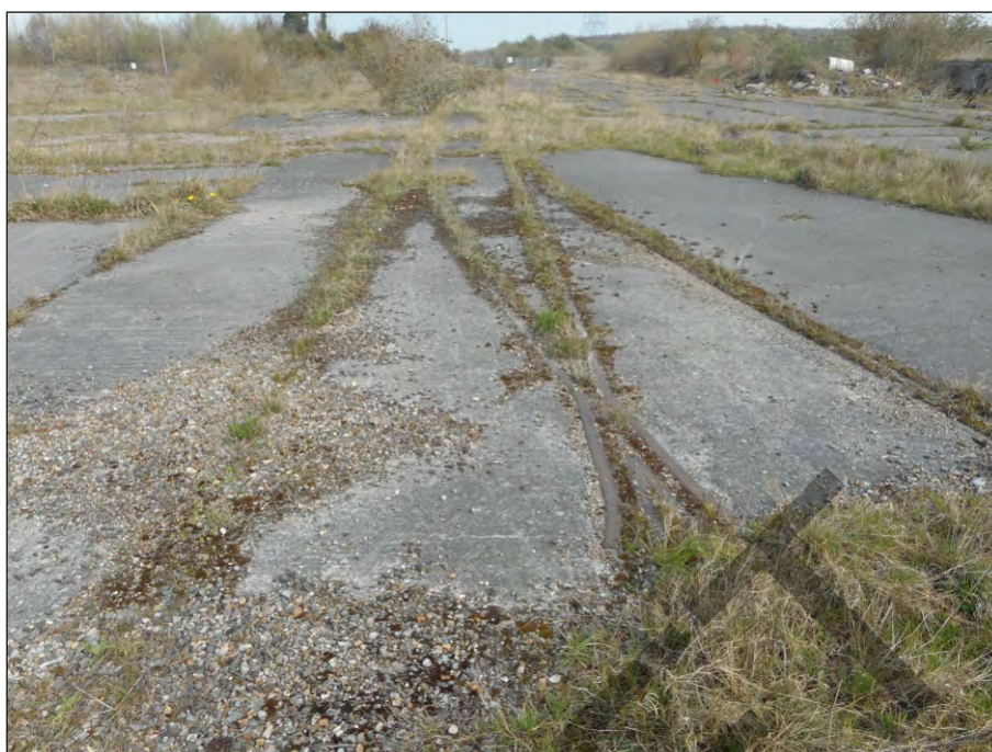
Plate 17: Section of tramline within the Site (WA663)
