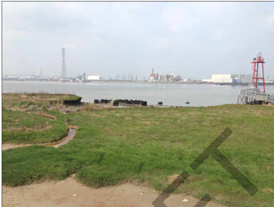
Plate 21: Anti-tank blocks on the foreshore (WA776)
