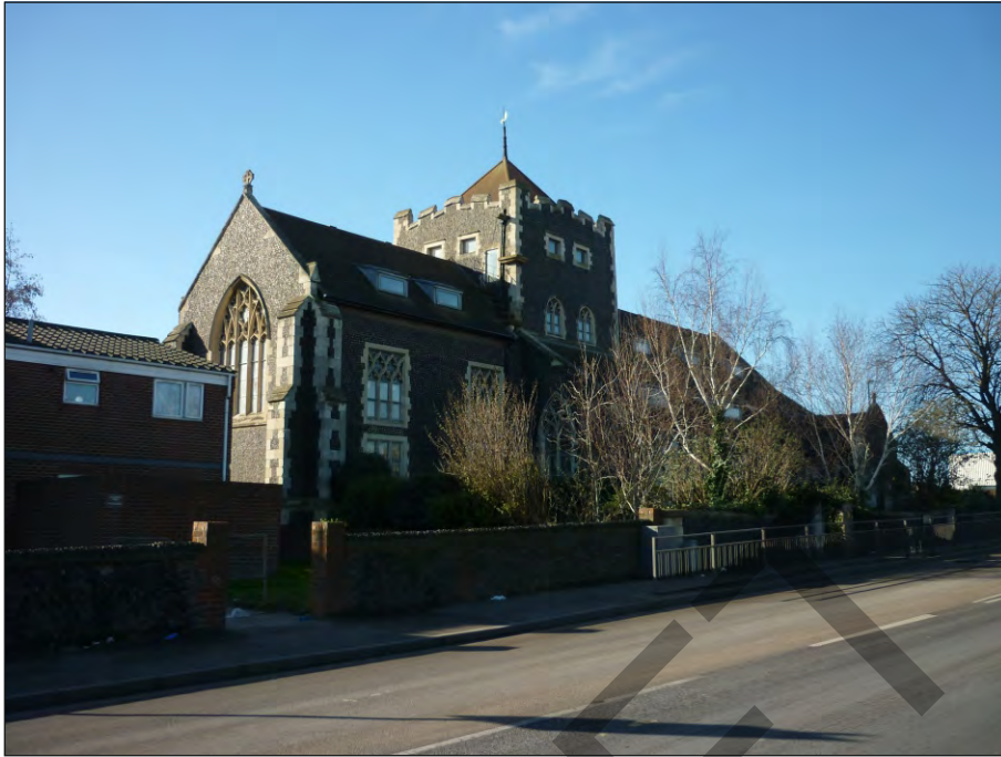
Plate 7: View of All Saints Church (WA647) within the Site
