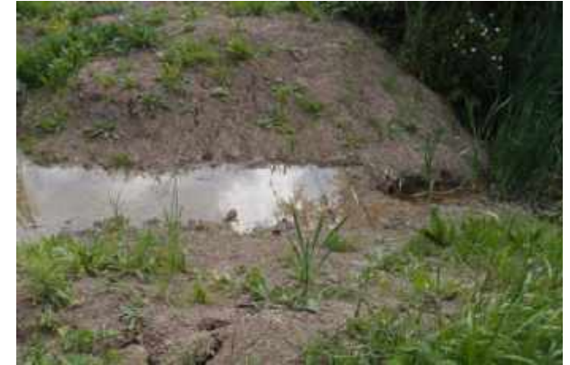
Photograph 30 Ditch outfall from New Pond.
